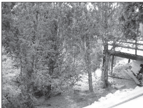
This home in Pocatello, Idaho, was surrounded by trees that were too close to the structure, which made it vulnerable to wildfire.
