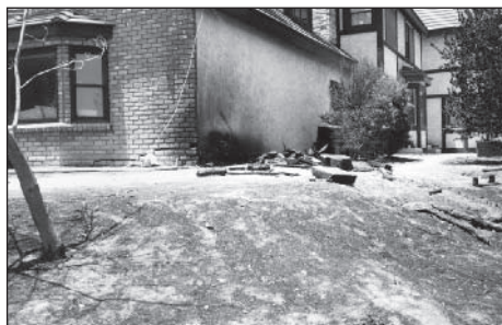
This house in Santa Barbara, Calif., was able to survive a wildfire because of a combination of brick and stucco siding construction with double-paned windows and the creation of a defensible space.
